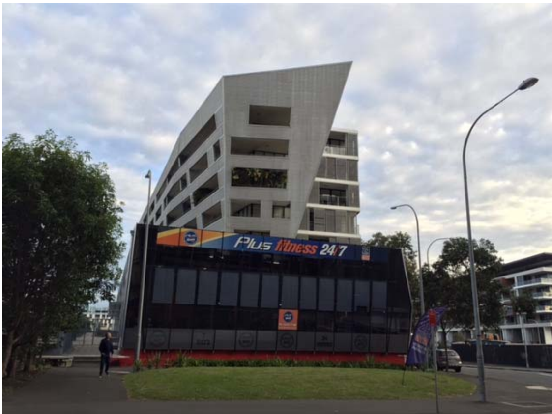
Figure 4: Alpha G development to the west of the site at 11A Lachlan Street
