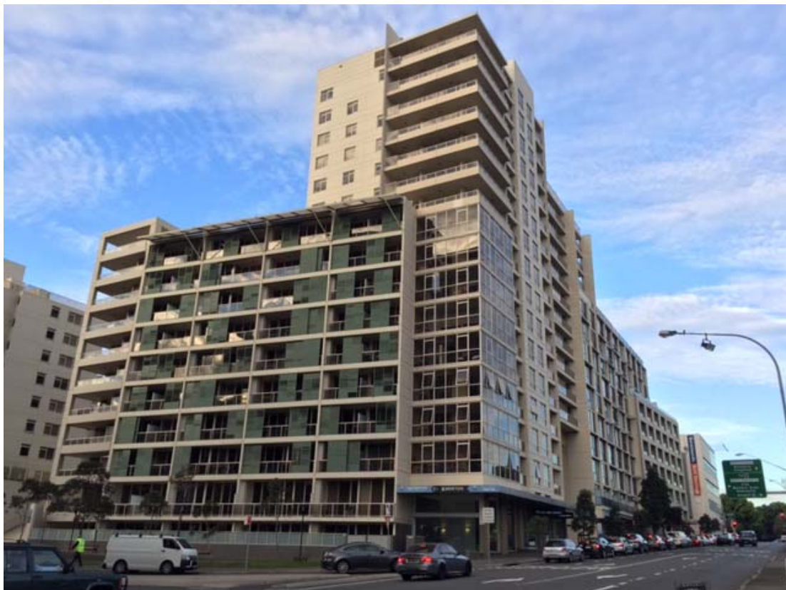
Figure 8: The eastern side of the Crown Square development at the corner of Lachlan and South Dowling Streets
