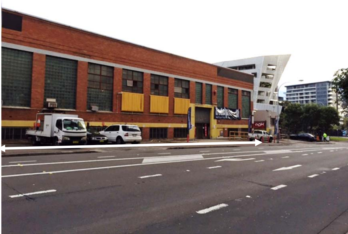
Figure 3: View along Lachlan Street looking west
