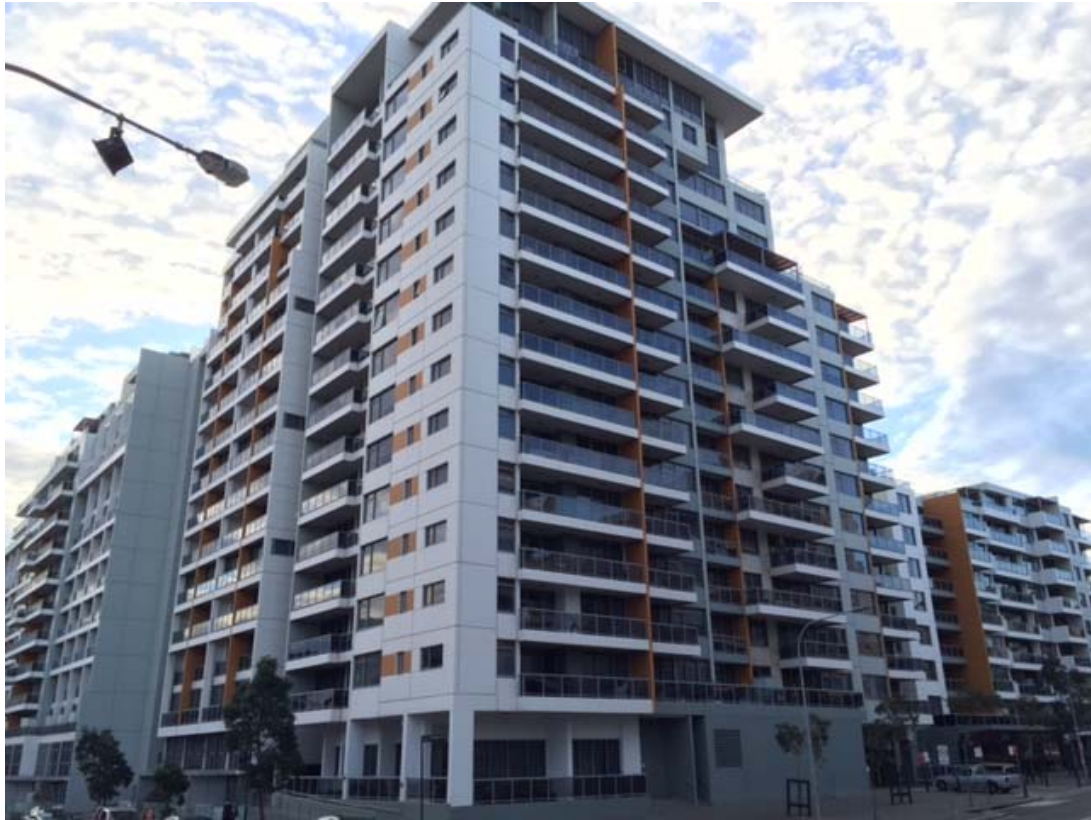
Figure 7: Crown Square development to the north on the opposite side of Lachlan Street
